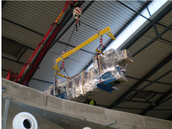
Fig. 13: The Linac is being lowered into the Linac bunker
