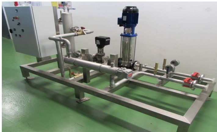
Cooling rack for HOM temperature tuning
