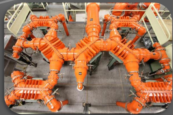
4 stages of 3 dB hybrid coaxial combiners (as already existing)
